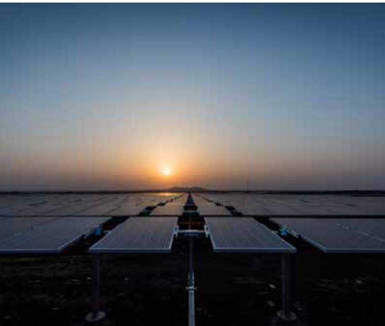
A solar power plant near Hyderabad, constructed with the assistance of Chinese enterprises.
