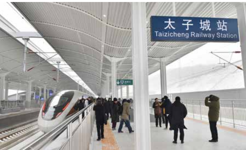
A high-speed train arrived at Taizicheng Station in Chongli District of Zhangjiakou, north China's Hebei Province, on December 30, 2019
