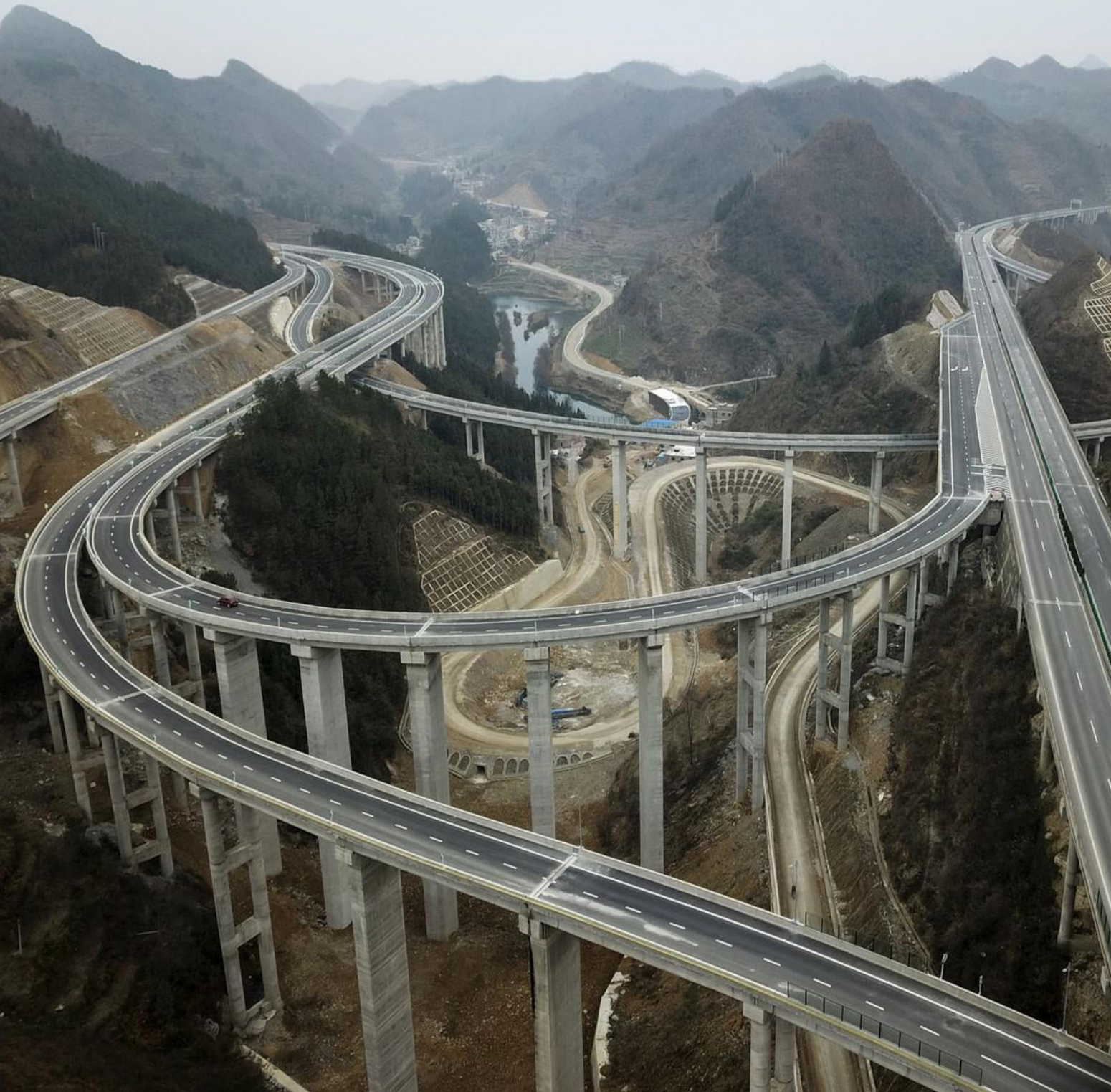
An aerial view of an intricate interchange on the Anshun-Ziyun Expressway, China
