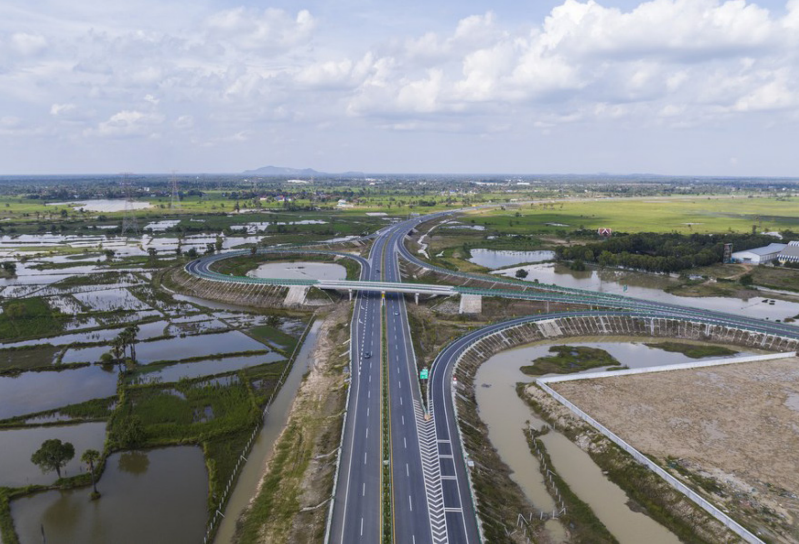
Cambodia's Golden Port Expressway in Kampong Speu province.
