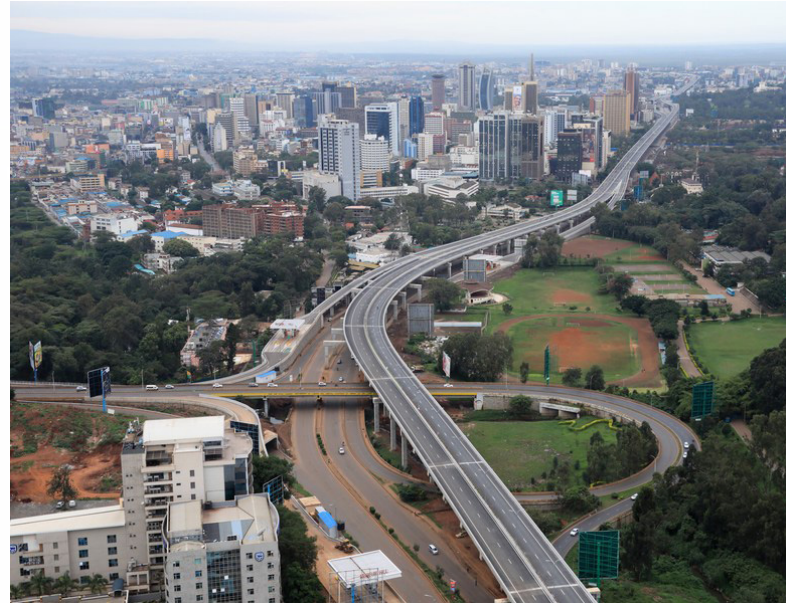
A section of the Nairobi Expressway built by China Road and Bridge Corporation in Nairobi, Kenya.
