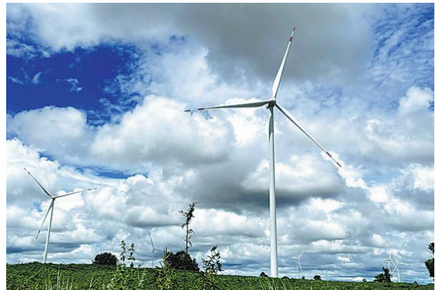
The wind turbines provided by China's Goldwind generate power in Chaiphum, Thailand.
