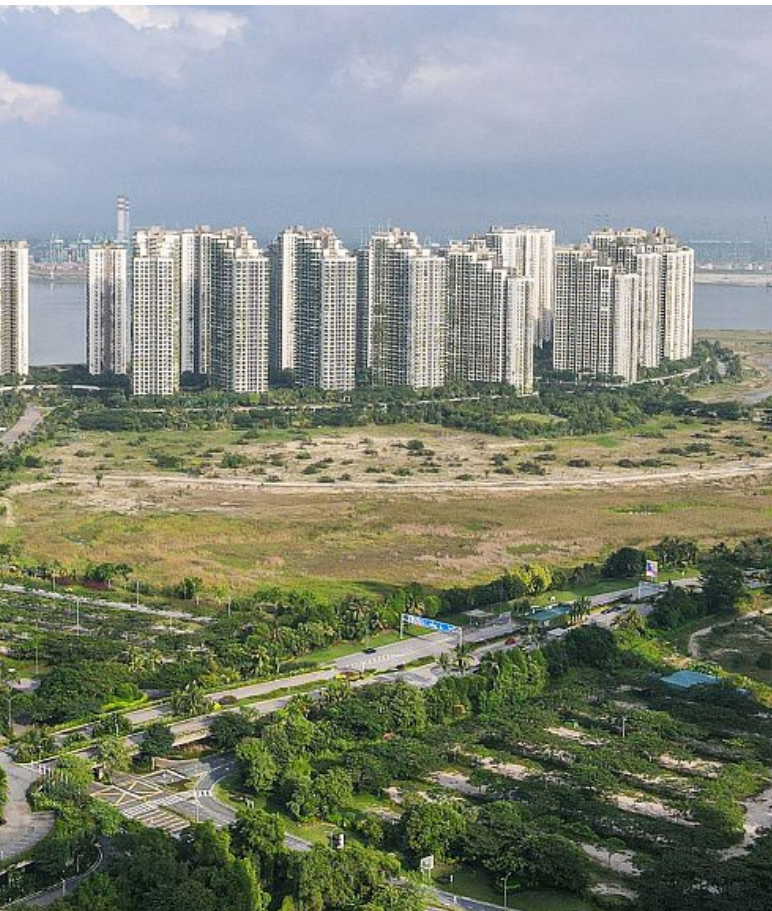
A general view of Carnelian Tower (L) and condominiums at Forest City, a development project launched under the Belt and Road Initiative, in Gelang Patah, Malaysia’s Johor state.
