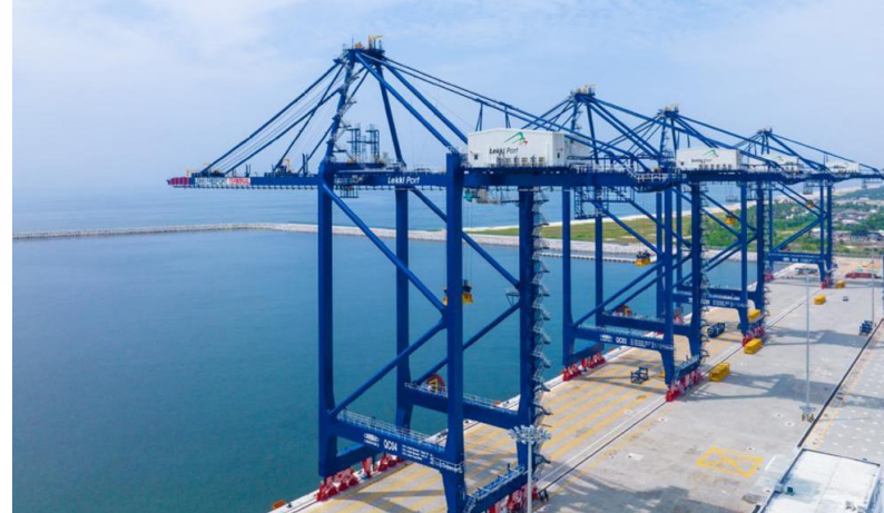
Facilities at the Lekki deep seaport in Lagos, Nigeria.
