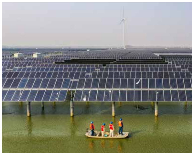
Electricity workers patrolling amid a photovoltaic and wind power generation project installed above the fishery waters in Sheyanghu Township of Baoying County of Yangzhou, east China's Jiangsu Province.
